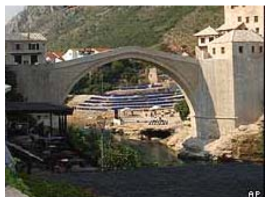
The reconstructed bridge
